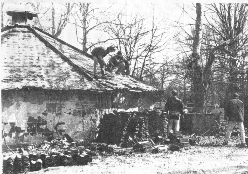
Maintenance workers removing tiles from the Ice House.
